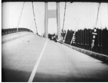
Figure 1.1: A famous example of the consequences of stretching models beyond their limits: The Tacoma Narrows Bridge collapsing because of driven oscillations in moderate winds. Also a stretch of association.
